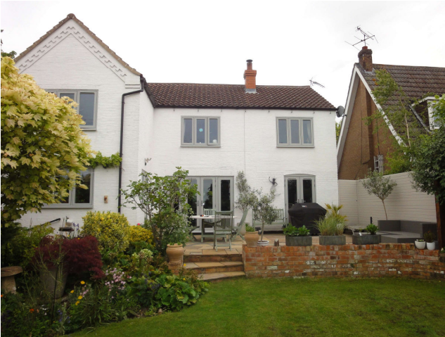
Patio area before construction has commenced
