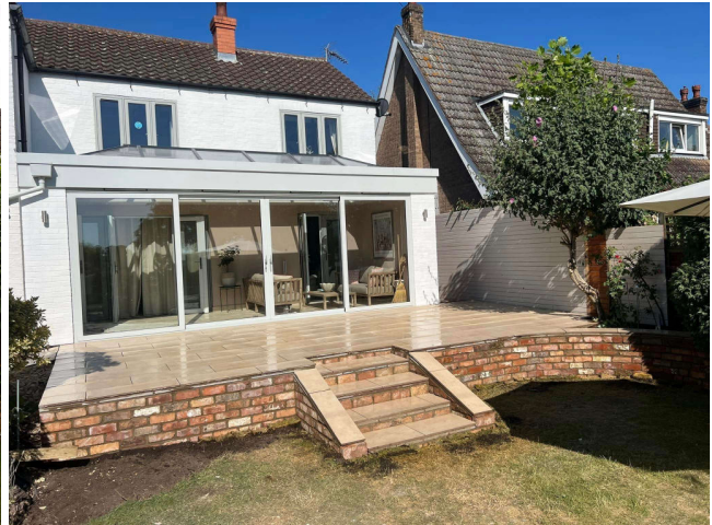
Patio area after we have left site
